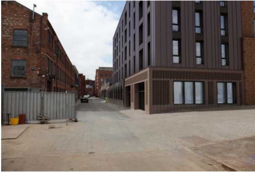
View 3: Looking west along Jersey Street
