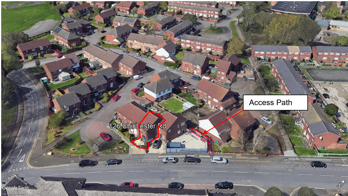
Image 1 Aerial View to show relationship between the application site (edged in red) and neighbouring properties. Source: www.google.com/earth
